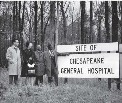
Site of Chesapeake General Hospital, which Opened in 1976 Credit: Chesapeake Regional Healthcare
